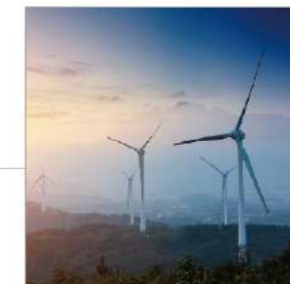
Wind power generation
